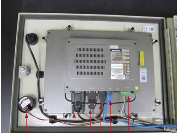
Figure 1: Interior of Door
