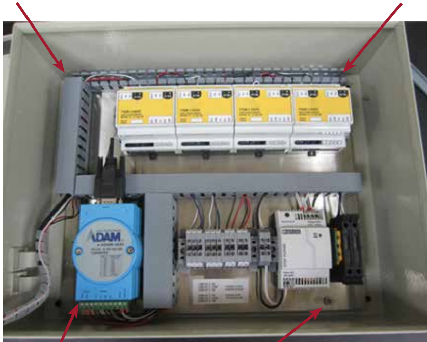
Back plane assembly securing bolt locations
